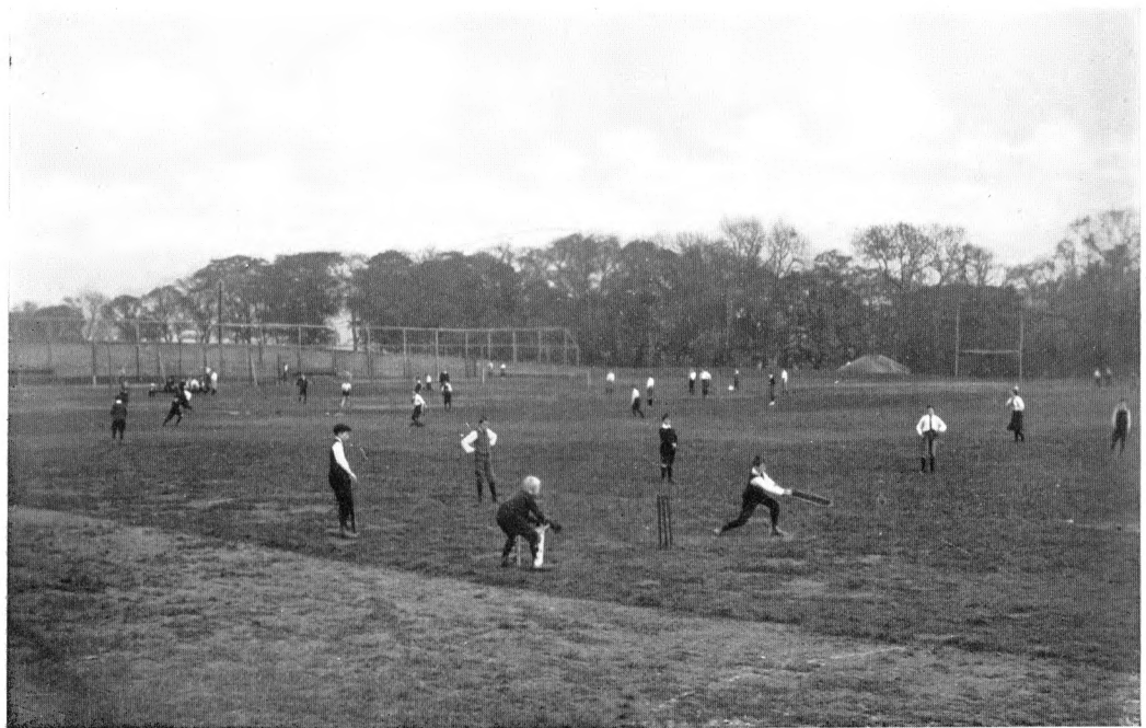
HIGH SCHOOL, RECREATION GROUND.
