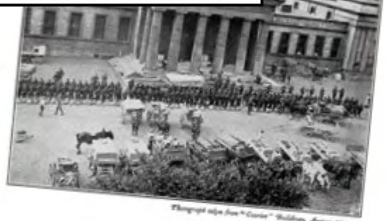
Photograph taken from "Courier" Buildings August 1914
